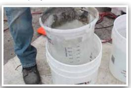
**3.** Pre-measure between 1.3 –1.6 gallons of water to 50lbs of Elephant Armor®. Vertical applications require less water than horizontal applications. *Never mix Elephant Armor® Primers as a liquid replacement into the mix.*
