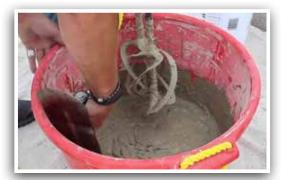
**5.** Trowel any unhydrated Elephant Armor® from the side and the bottom of the mixing bucket, continue mixing for an addition 30 seconds.
