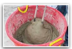
**7.** Add the balance of the water and continue mixing to achieve desired slump. Once the Elephant Armor® has been completely mixed to its desired slump, it will begin to set quickly. Additional water will not retemper the mix.
