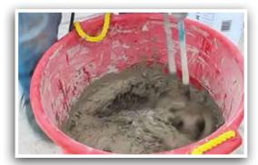
**6.** Make sure all material has been completely hydrated and mixed. This will ensure a homogeneous mix providing maximum performance of the Elephant Armor®.
