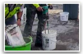
**8.** After mixing is complete, immediately submerge paddles into a bucket of water and run mixer to remove all excess Elephant Armor® from the paddles. Excess material left on the paddles will be extremely difficult to remove. Impact cleaning will damage paddles.
