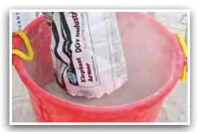
1. Vibrations during transport may cause clumping and compaction. Tap or roll the Elephant Armor® bag in the same manner you would soften a bag of ice. Pour Elephant Armor® into a 70 qt. mixing bucket.
