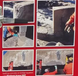
Sealing concrete on bridge repaired with Elephant Armor DOT
